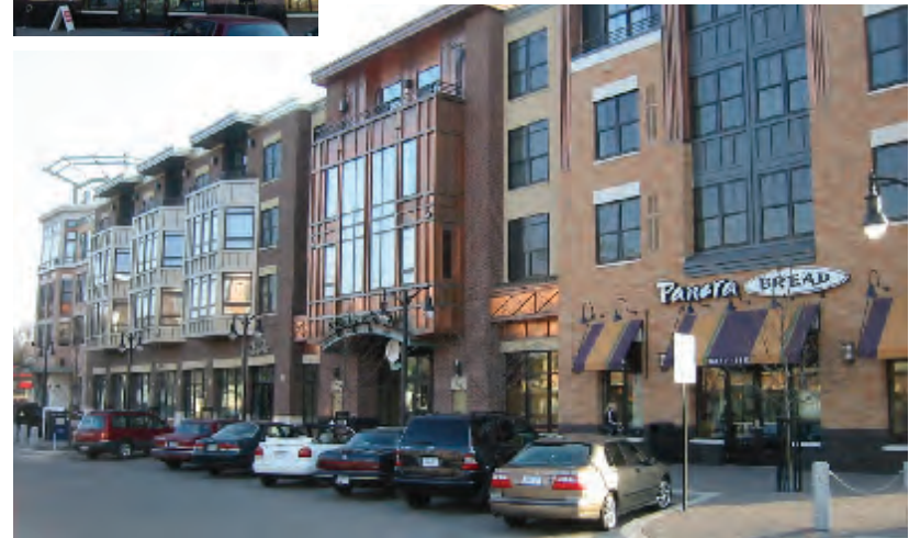
Multi-story buildings shall have the ground floor distinguished by intermediate cornice lines or other architectural detailing as shown
