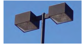
Shoe-box lighting or other downcast fixtures to be used in large parking areas
