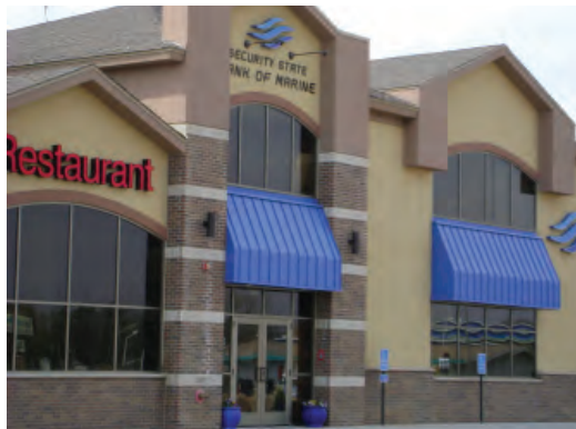
All building fronts must include four elements such as 30% first floor window coverage, irregular building shapes, architectural detailing and contrasting colors
