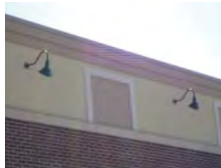
Wall mounted lighting shall be used to illuminate entry points and highlight architectural features
