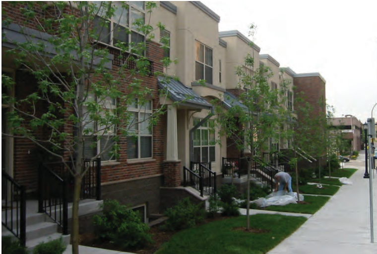
The first floor elevation shall be minimum of 2'-6" above the sidewalk immediately adjacent to the front of the unit to ensure the unit is raised from the public space
