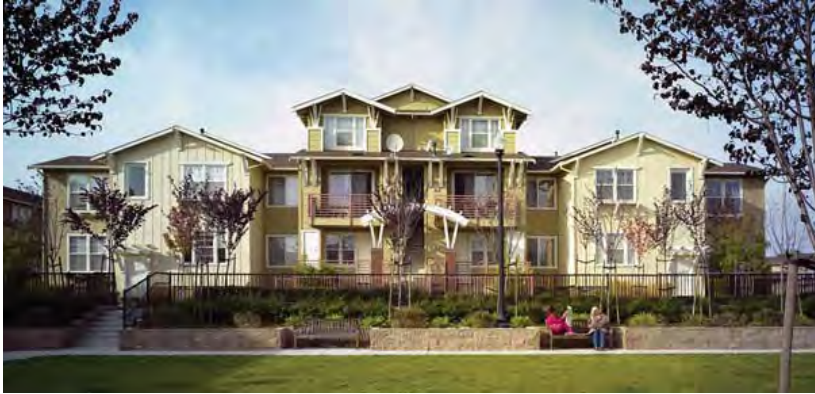
Building and roofing materials shall meet current accepted industry standards
