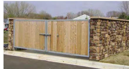
Any trash enclosure shall be constructed of the same materials as the principal building
