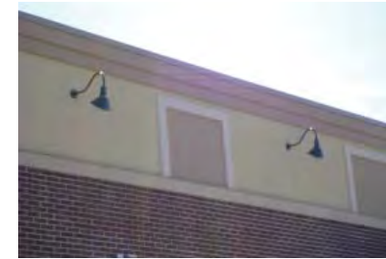
Wall mounted lighting shall be used to illuminate entry points and highlight architectural features
