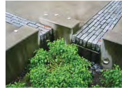
Water collection systems integrated into pavement areas
